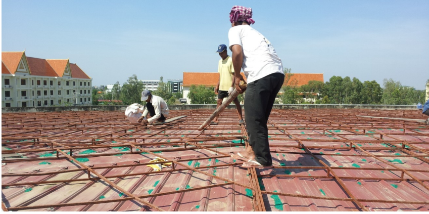
Laborers work on the roof of the courthouse in preparation for the upcoming rainy season during the trial recess, which ended on 9 March.
